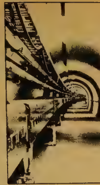
Bending magnets in interior of Main Accelerator at National Accelerator Laboratory. The Main Accelerator is four miles in circumference; 1.24 miles in diameter. NAL Photo.
